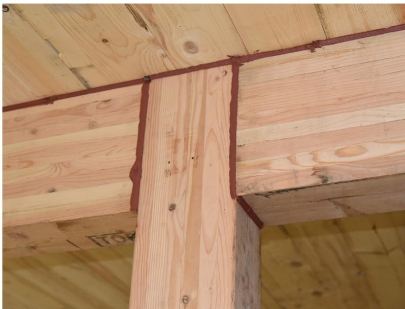
**Figure 7-2.** In buildings of Type IV-A, IV-B and IV-C construction, IBC Section 703.7 requires that sealant or adhesive be provided to prevent air flow at intersections of panels, beams and columns. The sealant or adhesive would not normally be seen protruding from intersections as shown here.
